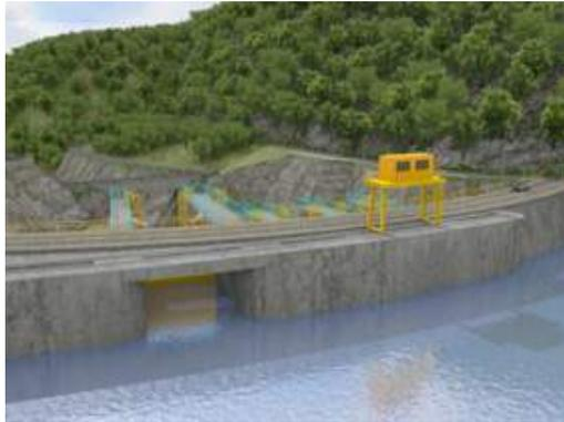
The hydropower plant is designed as run-of hydro just like micro hydro where the operations are adjusted to the water level in the river. Run-of hydro does not hold water like in reservoir hydropower plant, it uses the natural stream. Water reserves are not stored in the reservoir but stored naturally in the upstream forests of Batang Toru watershed.
